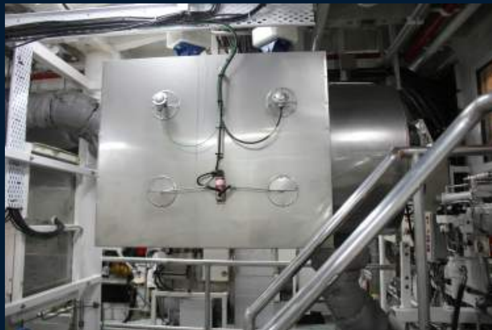
Engineer, procure and install soot elimination system
